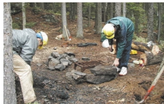
Installing a campsite fire grate.
